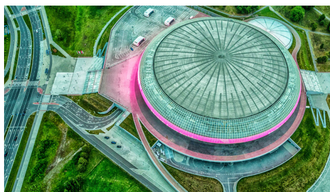
TAURON Arena Kraków
